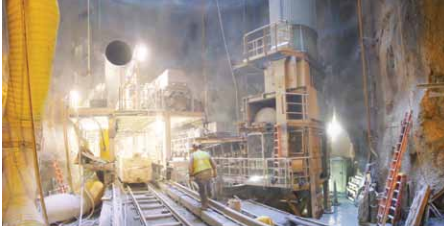
200 feet below ground, workers have begun excavation of the 3-mile long storage tunnel.
